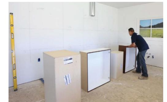
5. It is best when installing a larger kitchen to mark the cabinet positions and code (size) on the wall. Better to find out now if things aren't going to fit just right than after you've installed several cabinets.
