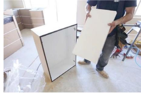
7. Remove all doors, drawers and shelves, being careful to mark them so that they go back on correct cabinets. Removing the doors can be done without tools as the hinges are "clip-on".
